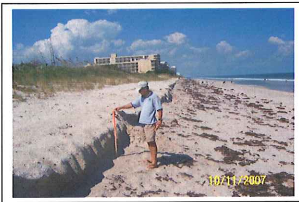
Figure 1: Surveying Mid Reach Erosion
